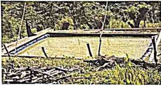
A water harvesting tank constructed on hill slopes Plantation for conservation of top soil nutrients
